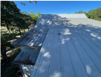
4. – 6. Sample of 24 gauge, double lock, standing seam to be painted in option #1 – Patina Green
