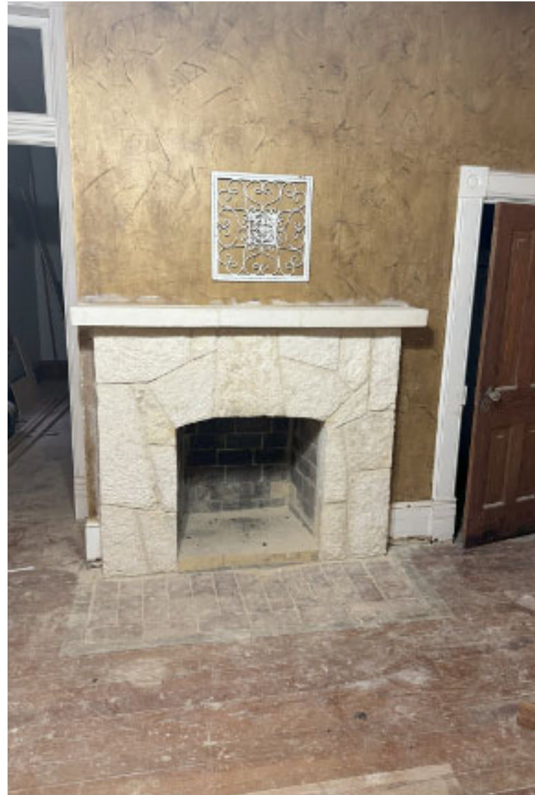
Existing fireplace in parlor, existing wood floor uncovered from 4 layers of material including concrete.
