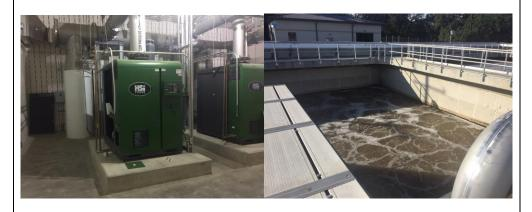
However, we started having operational issues with two of the units. It was determined that the way their output was being reduced due to the current size of the plant was harmful. We have changed our operations to minimize this wear and tear. However, we now have equipment that is in need of repair.
