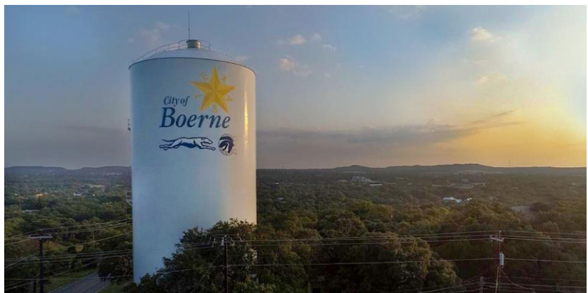
Figure 7. A City of Boerne water tower
