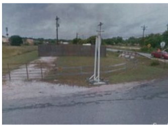
School Lift Station
