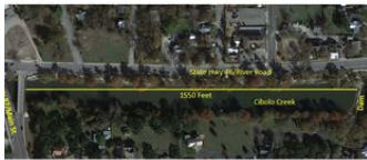
River Road Park aerial
