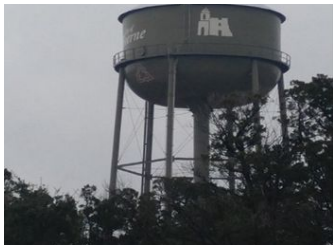
Reclaimed Water Elevated Tank
