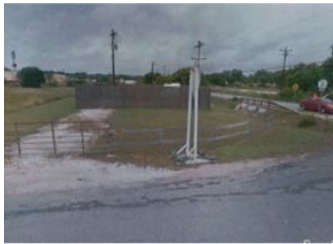
School Lift Station
