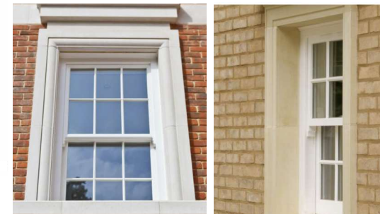
CAST STONE JAMBS/HEADERS AND SILLS
