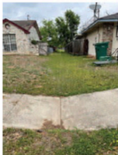
Existing outfall through two residential properties of drainage area to Cibolo Crossing Subdivision.
