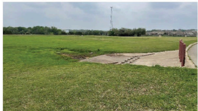
Location of proposed inline extended detention basin to limit downstream sedimentation and floatables transferred downstream.
