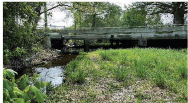
Existing bridge crossing at Cibolo Creek and Herff Road.
