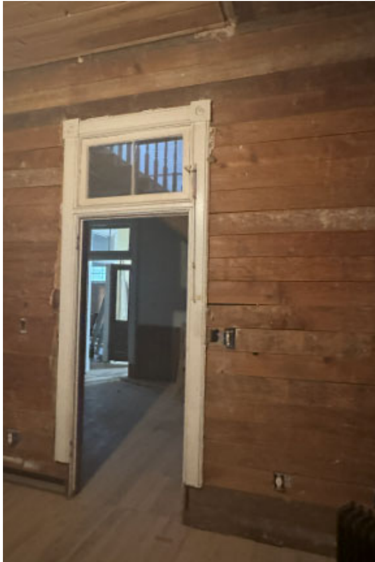
Typical door opening with original wood plank walls, this was covered with wall paper and then sheet rock.
