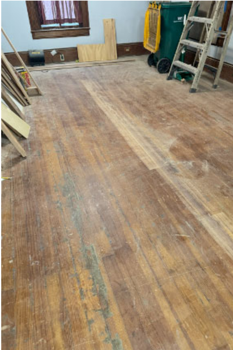
Existing wood floor exposed from under parquet floor.
