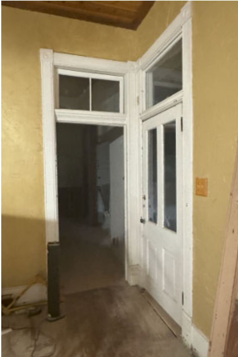
Typical interior doors and transoms.
