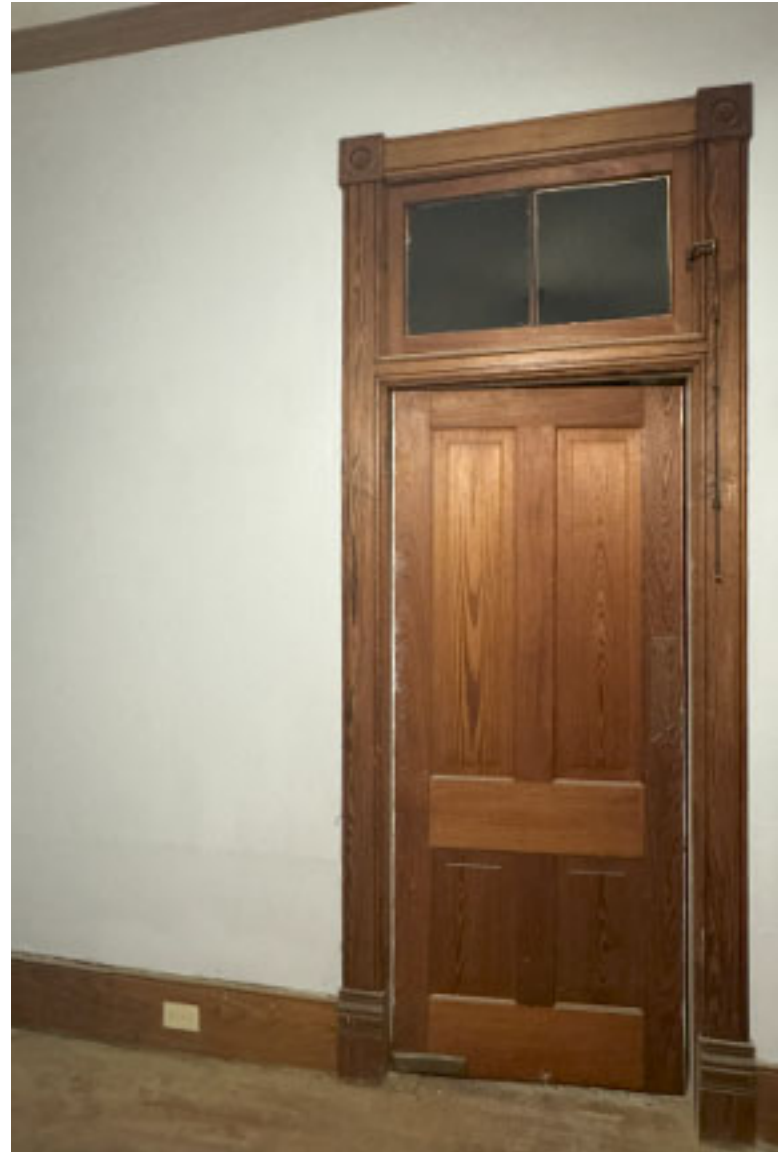
Typical original door and glass transoms.
