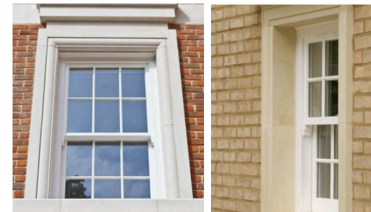
CAST STONE JAMBS/HEADERS AND SILLS
