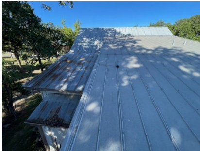
4. – 6. Sample of 24 gauge, double lock, standing seam to be painted in option #1 – Patina Green
