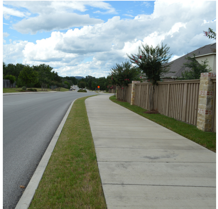
The existing Lattimore Boulevard sidepath extends for almost a half-mile, and serves as an example of a facility that connects users of all ages within a neighborhood.
