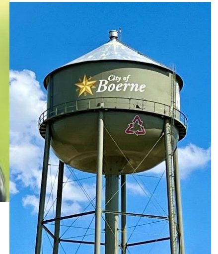
Reclaimed water tower at Esperanza
