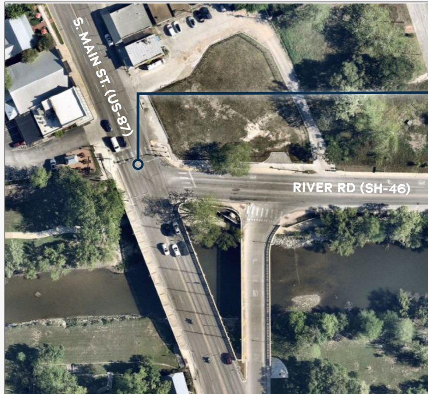
Figure 6.2: Main St & River Rd (SH-46)
